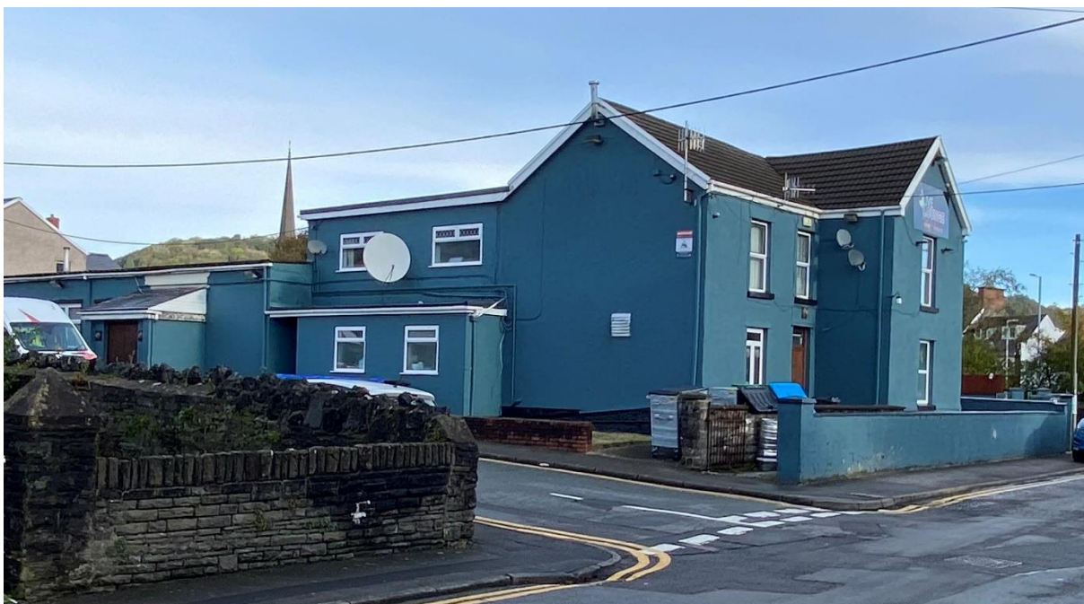
View of premises at junction of Ynisderw Road and Francis Street, Pontardawe Page 257
